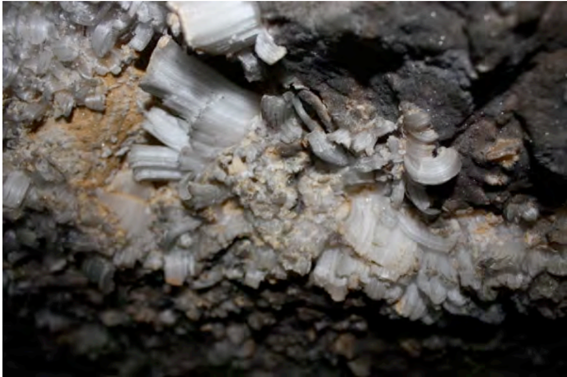
Salt crystals that have formed on a wall in the substructure of the Step Pyramid.
